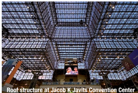
Roof structure at Jacob K Javits Convention Center
